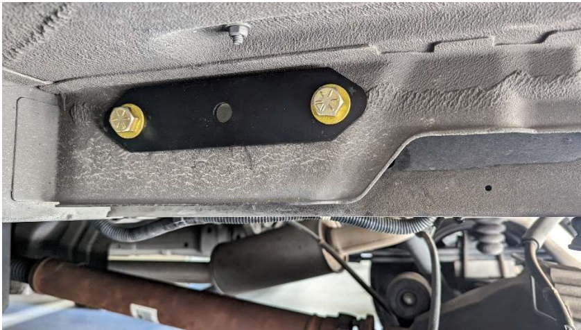
After Installing reinforcement plate
